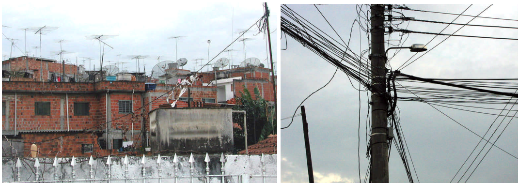
Figure 1. A view of Heliópolis (left), and the pole with illegal energy connections (right)
